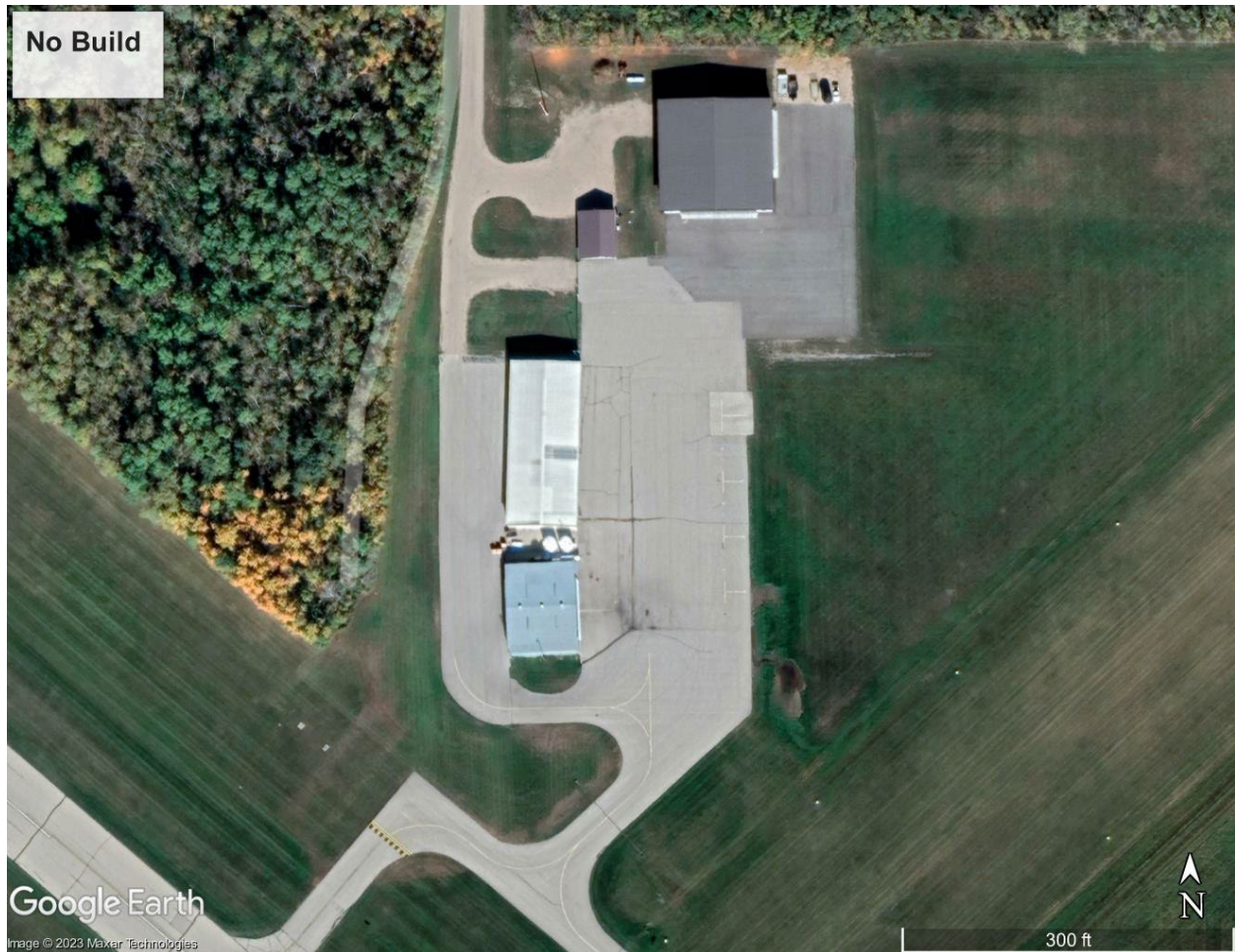
Figure 5-2 - Existing Terminal Area
